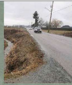
Looking NB on Prest Rd From 6B-A-34-B
